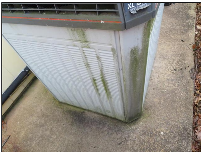
8.8 Item 10(Picture) Clean algae off of the air condenser
