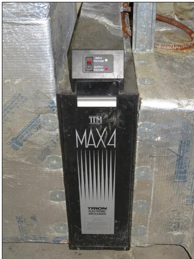
8.15 Item 1(Picture) Electronic air filter
