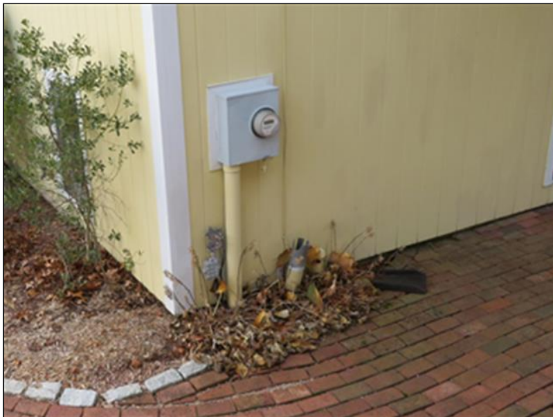
12.8.B Item 2(Picture) Electric meter for main and sub panels
