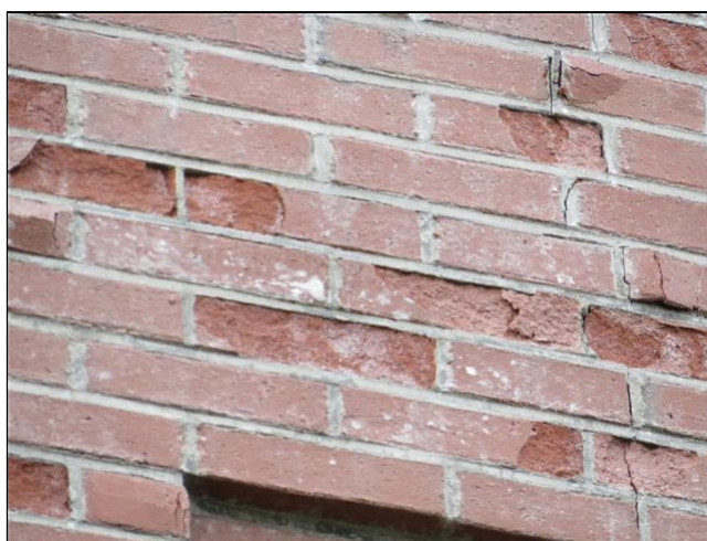
1.14 Item 4(Picture) Spalling bricks
