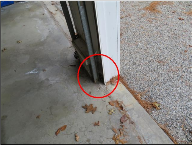
3.19 Item 3(Picture) No electric eye for middle door
