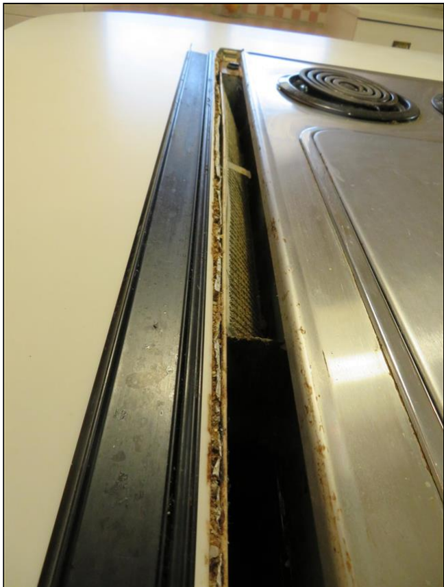
10.8 Item 5(Picture) Clean or replace filters
