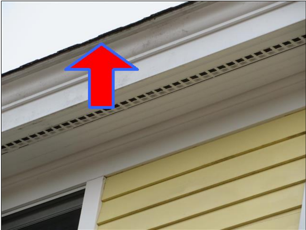
1.3 Item 1(Picture) Recommend installing gutters.
