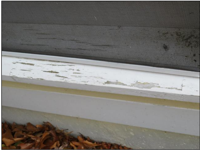
2.2 Item 1(Picture) Scrape, sand, prime and paint window sills.
