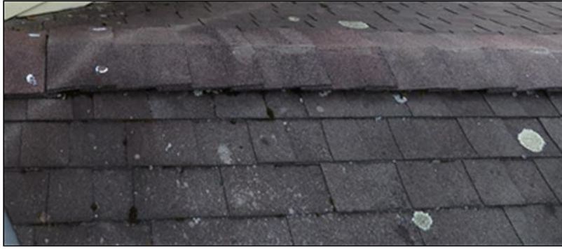
1.13 Item 1(Picture) One layer of architectural roof shingles
