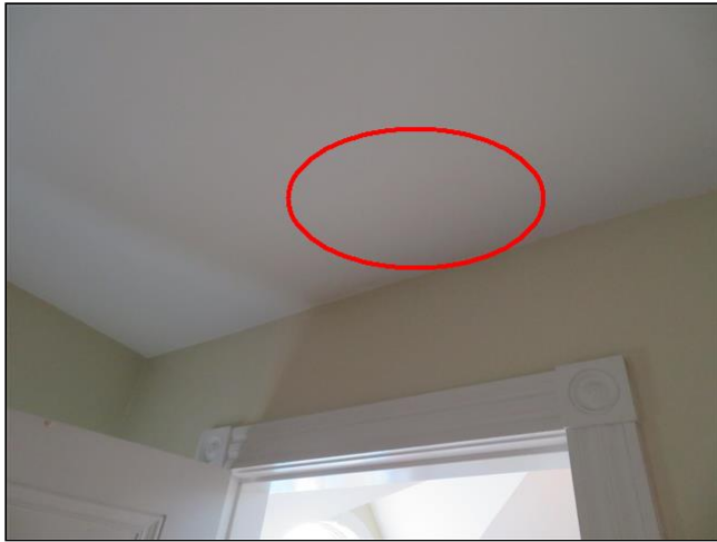
7.8 Item 3(Picture) Missing smoke alarms in bedrooms
