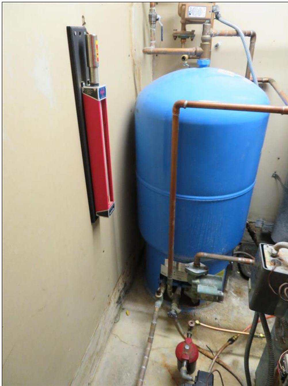
15.0 Item 1(Picture) Well holding tank
