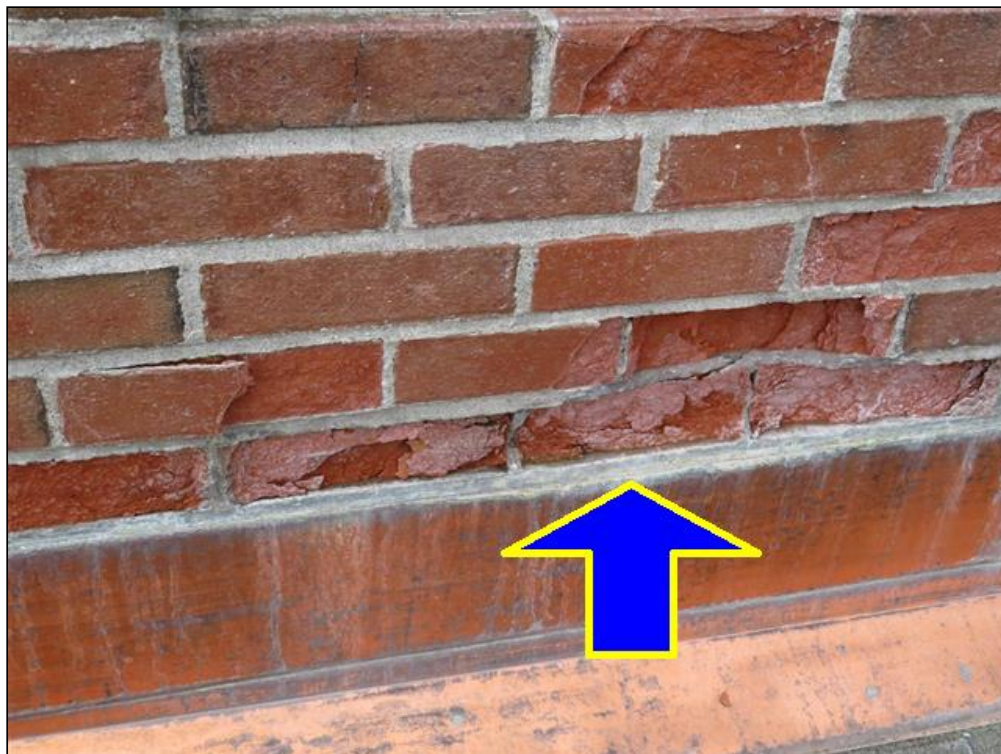
1.14 Item 2(Picture) Spalling above flashing
