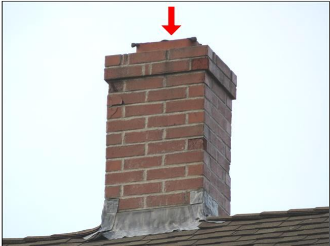
1.10 Item 1(Picture) Stainless steel rain cap recommended
