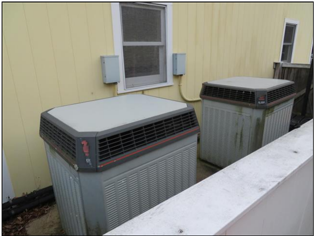
8.8 Item 3(Picture) Two air condensers on side of garage
