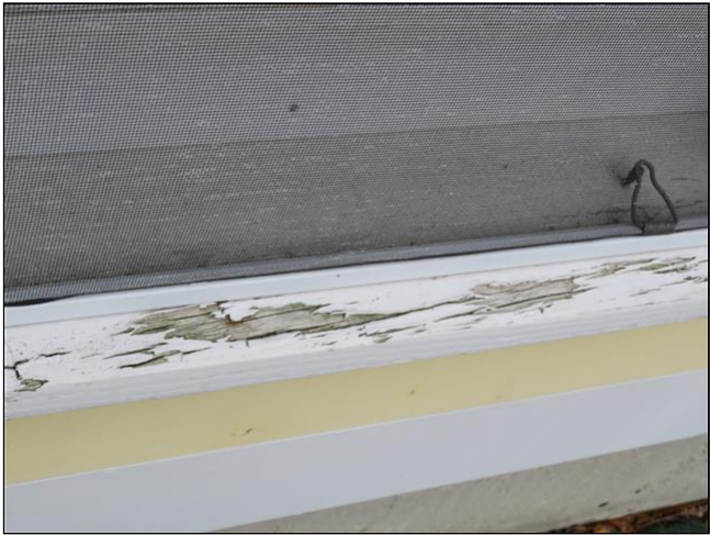
2.2 Item 2(Picture) Scrape, sand, prime and paint window sills
