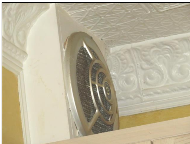
9.3 Item 5(Picture) The exhaust fan appears outdated
