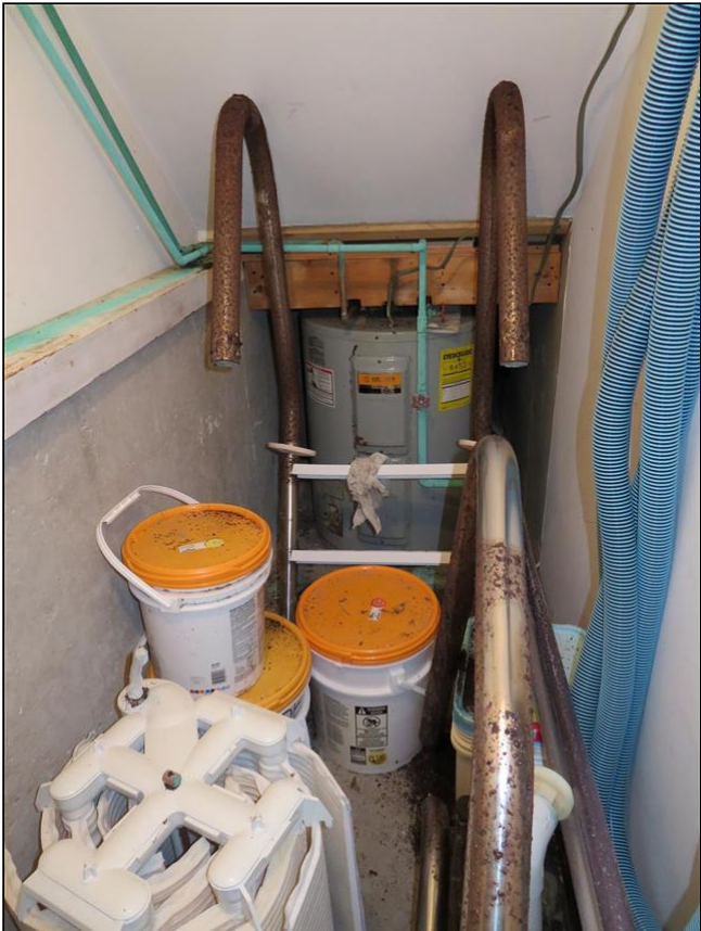
12.7.B Item 1(Picture) 29-year old, State brand, 40-gallon water heater
