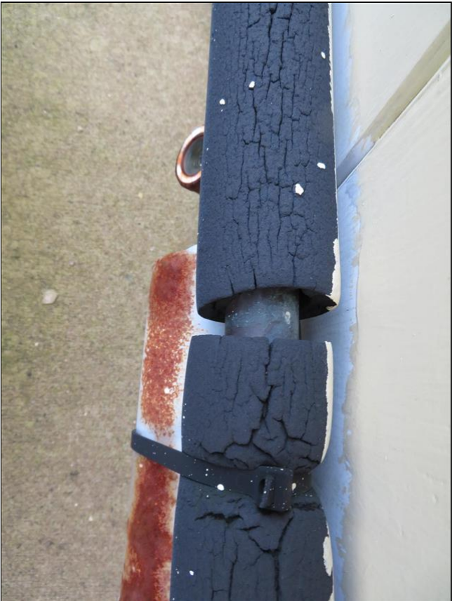
8.8 Item 7(Picture) Replace foam sleeves
