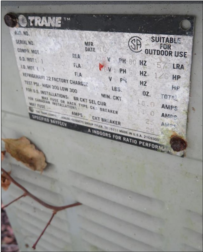
8.8 Item 2(Picture) Label serial number and manufacture date are illegible
