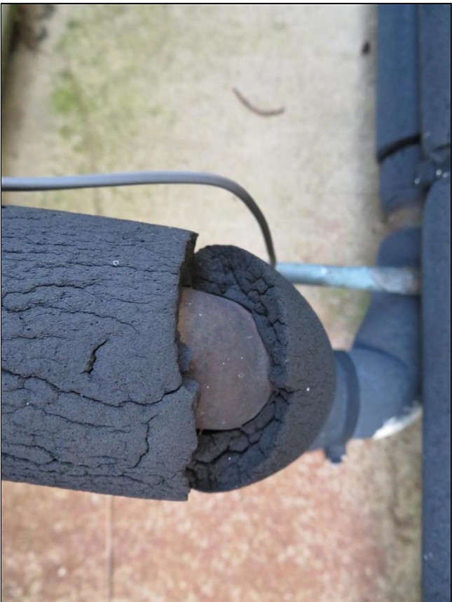
8.8 Item 9(Picture) Replace foam sleeves
