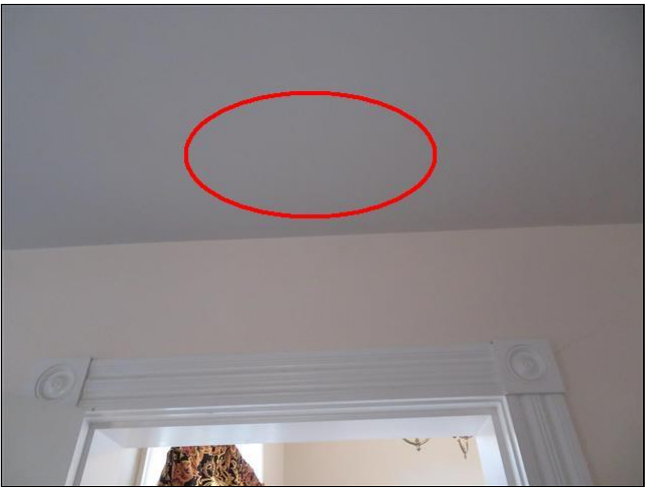
7.8 Item 2(Picture) Missing smoke alarms in bedrooms
