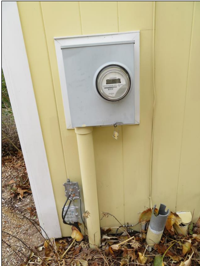
7.27 Item 1(Picture) One electric meter for both living quarters
