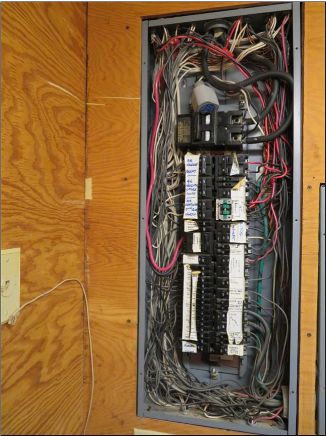
7.22 Item 2(Picture) Main panel with the cover removed
