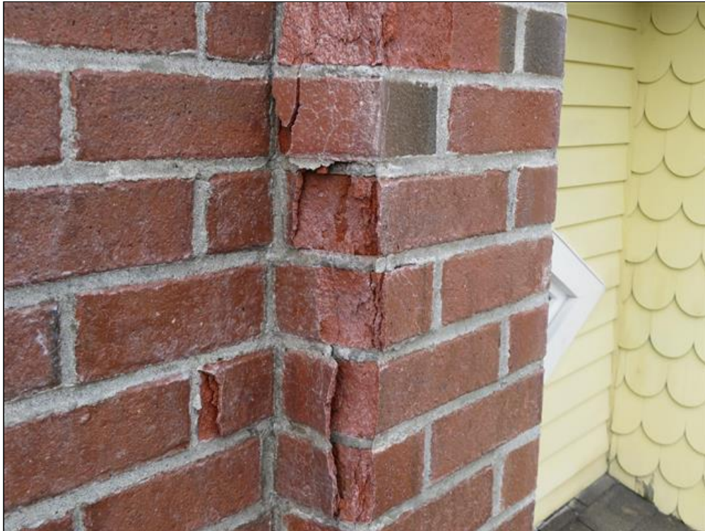
1.14 Item 1(Picture) Spalling bricks
