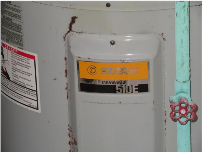
12.7.B Item 2(Picture) 29-year old, State brand, 40-gallon water heater
