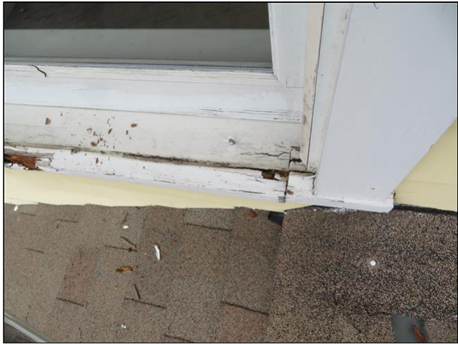
2.2 Item 3(Picture) Scrape, sand, prime and paint window sills.
