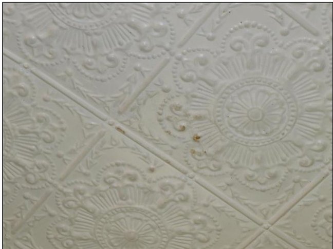
4.2 Item 1(Picture) Stains were observed on the kitchen metal ceiling
