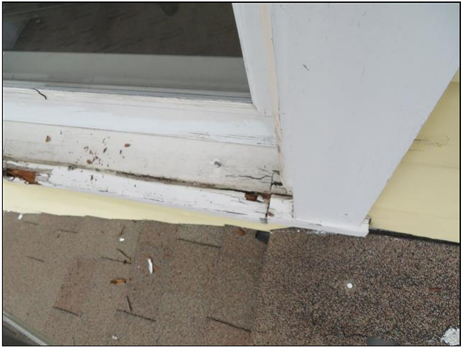
2.2 Item 4(Picture) Scrape, sand, prime and paint window sills.
