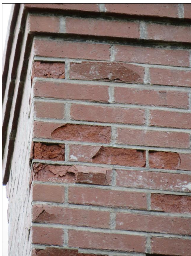
1.14 Item 3(Picture) Spalling bricks
