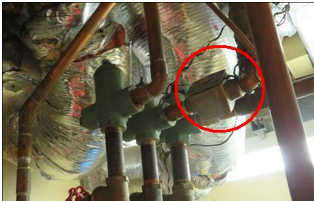
8.10 Item 1(Picture) Missing zone valve
