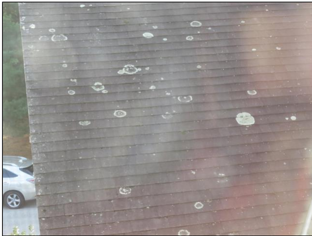
3.12 Item 1(Picture) Replace roof shingles
