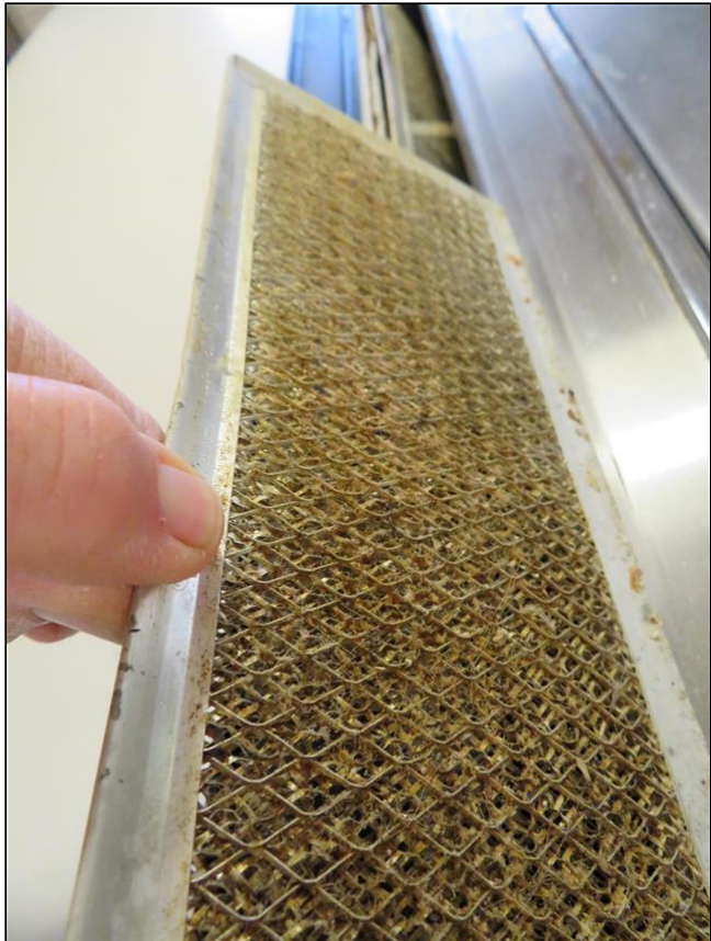
10.8 Item 3(Picture) Clean or replace filters
