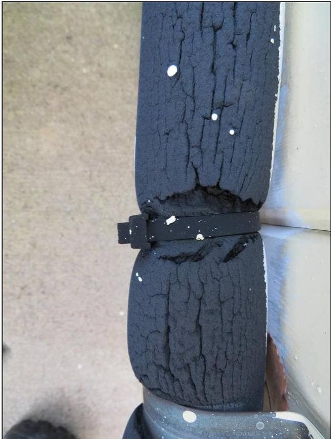
8.8 Item 6(Picture) Replace foam sleeves
