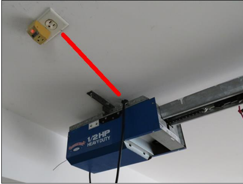
3.19 Item 4(Picture) Left garage door operator was not plugged into the receptacle.
