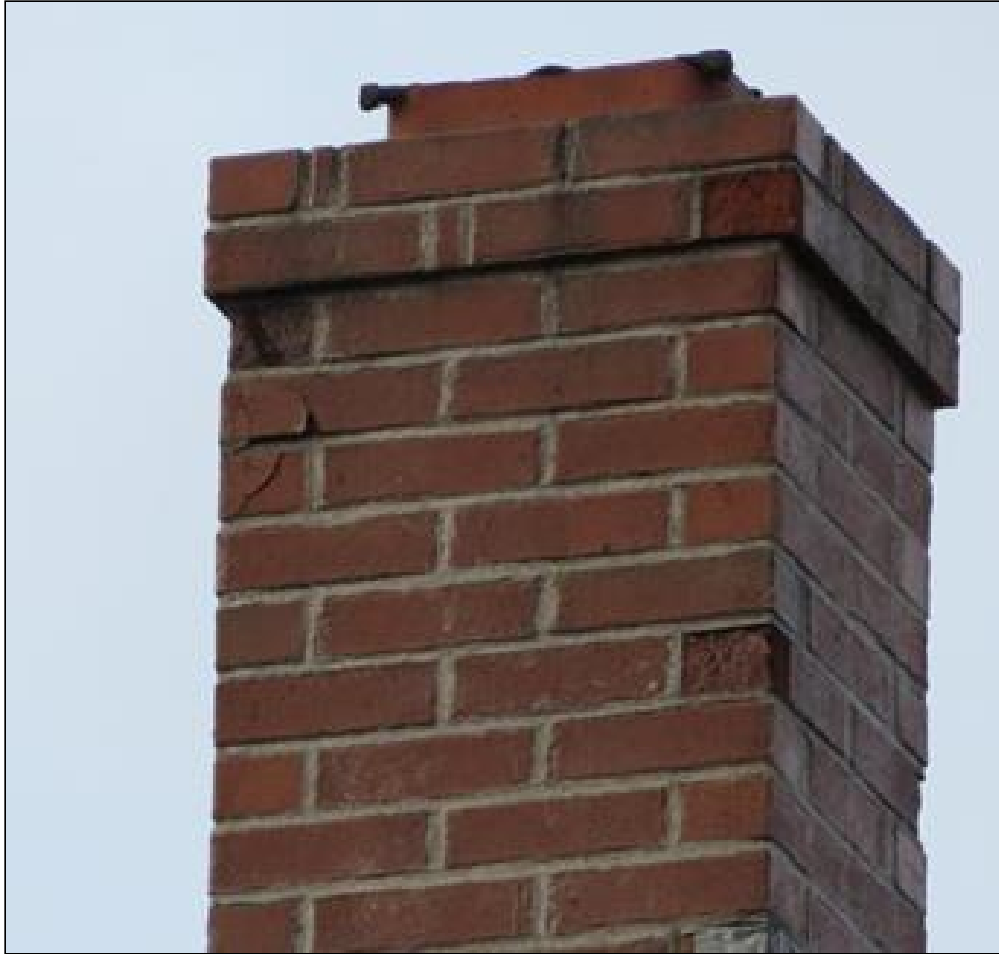
1.14 Item 5(Picture) Spalling bricks
