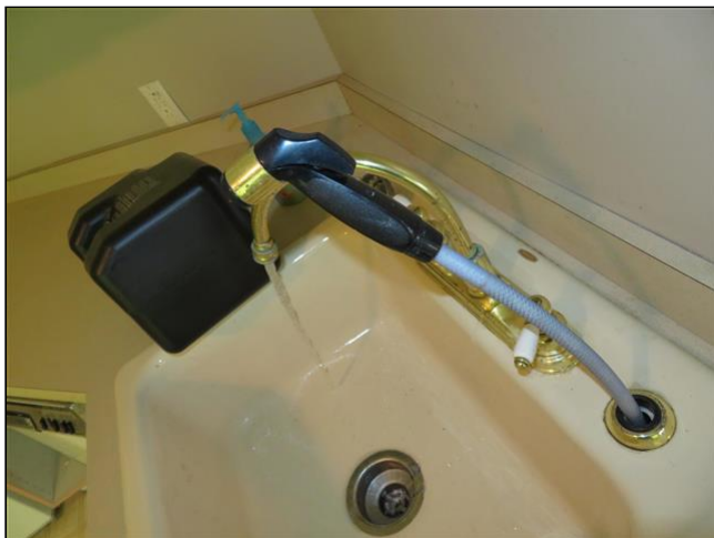
4.21 Item 1(Picture) Lower level kitchen sprayer was NOT operational
