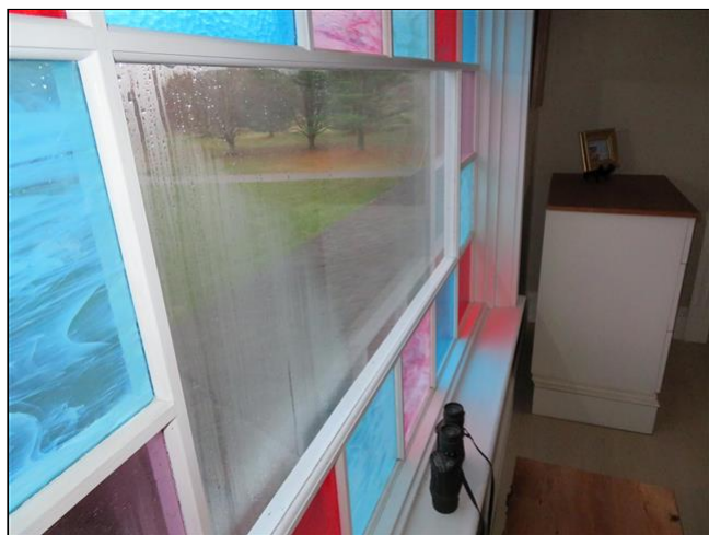
4.6 Item 1(Picture) Thermal leak
