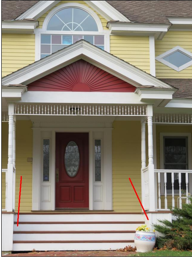
2.13 Item 2(Picture) Handrail is need at front porch steps
