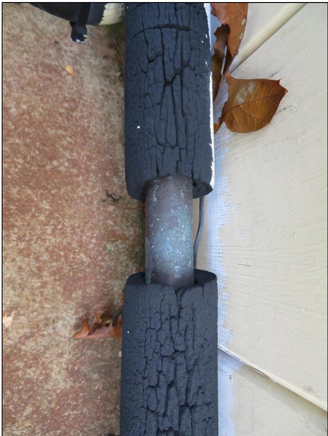
8.8 Item 8(Picture) Replace foam sleeves
