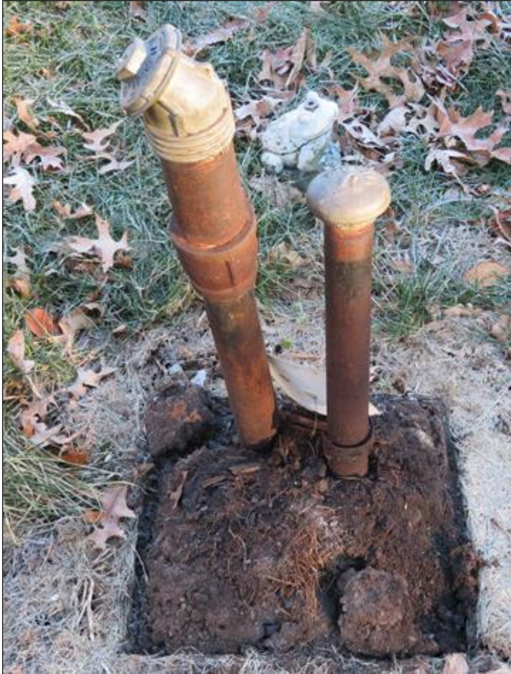
8.14 Item 4(Picture) Fill and vent pipes
