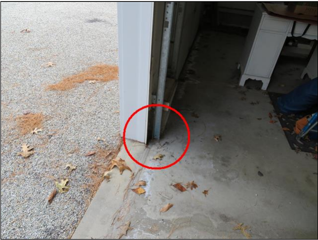
3.19 Item 2(Picture) No electric eye for middle door
