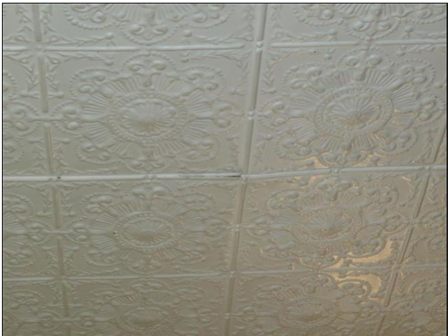
4.2 Item 2(Picture) Stains were observed on the kitchen metal ceiling
